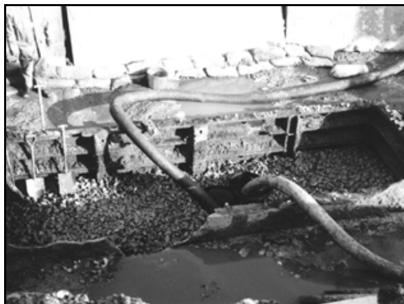
Figure 5. The shaft lining is exposed, dressed off and prepared for concrete
