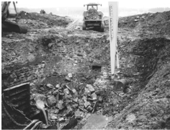
Figure 3. View of the excavation to intercept the Kames No. 1 shaft (located bottom left)
