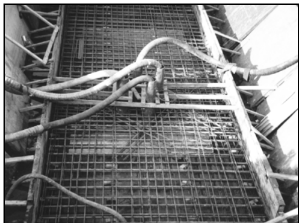
Figure 6. The shaft cap is prepared for the concrete pour; dewatering pipes in centre
