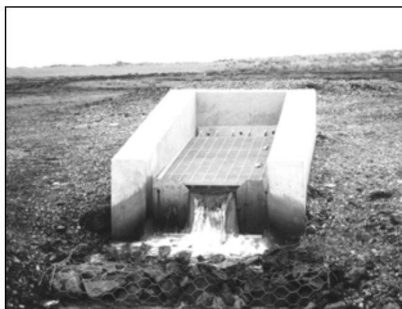
Figure 8. Finished mine water discharge point (the harness)
